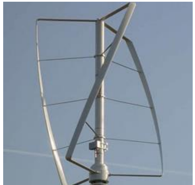
VAWT: vertical axis wind turbine
